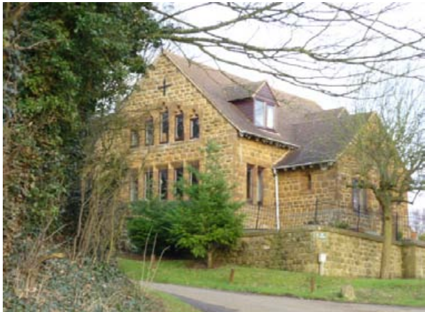
4 The National School building was constructed in 1872 of coursed ironstone. This is an ornate building that sits in an island in the carriageway on School Road now converted to a dwelling.
