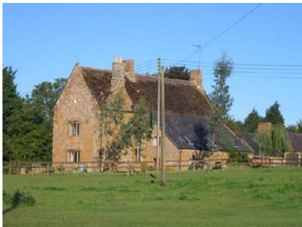
The later extension at Mansion House Farm has a Welsh slate roof
