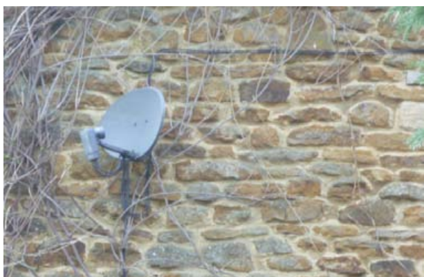
Satellite dishes on building frontages
