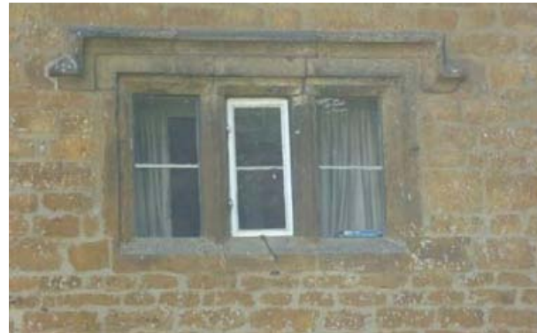
Stone mullioned windows at The Chestnuts
