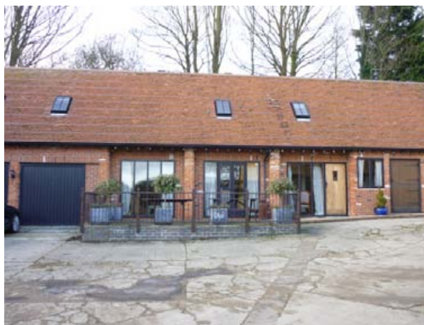
Single storey barn conversion at Church Farm
