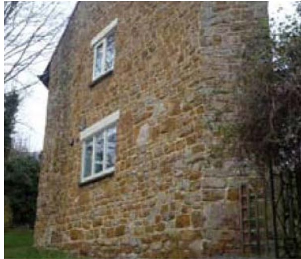
5 Sunnybank, an unusually formed building that sits aside Blacksmiths Lane at the heart of the village. The nature of the slope means windows are almost at ground level in places.
