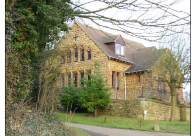
The conversion of the former Church of England National School into a dwelling has entailed splitting the fine trefoil gable windows and the insertion of a dormer window to accommodate an upper floor. The railings have been retained and the former use is still discernable, although the loss of the school bell is regrettable.
