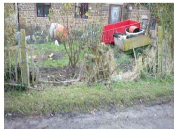
Loss of traditional means of enclosure has a negative effect on the streetscape
