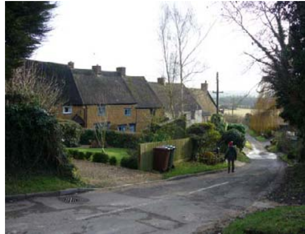
2 This terrace of cottages is not listed but are the best surviving example of 18th century labourers' cottages. Two storeys and constructed from coursed ironstone rubble they demonstrate the use of local building material in the construction of the most humble type of dwelling. The loss of original casements, the rendering of one cottage and car parking detract from this frontage which forms an important corner of the village green.
