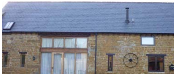
Welsh slate is now the predominant roofing material on older properties
