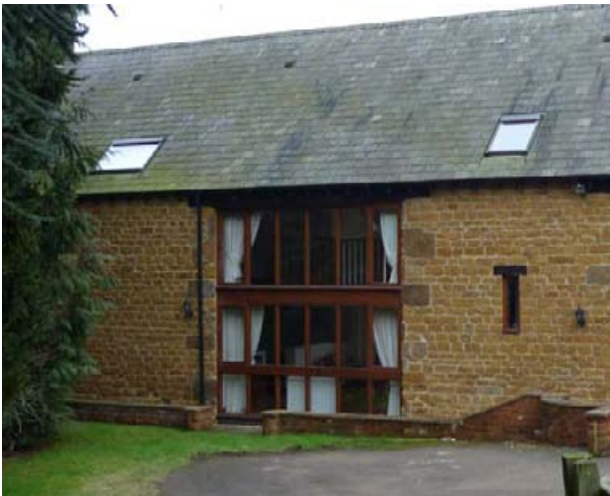
Former barn door opening retained
