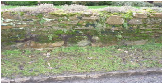
Occasional use of granite kerbing is unobtrusive
