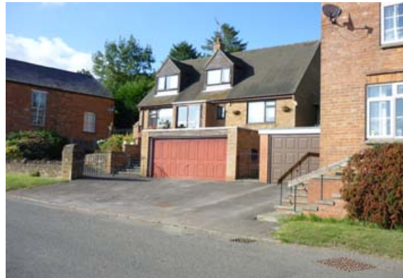
Buildings set back at western end of Main Street
